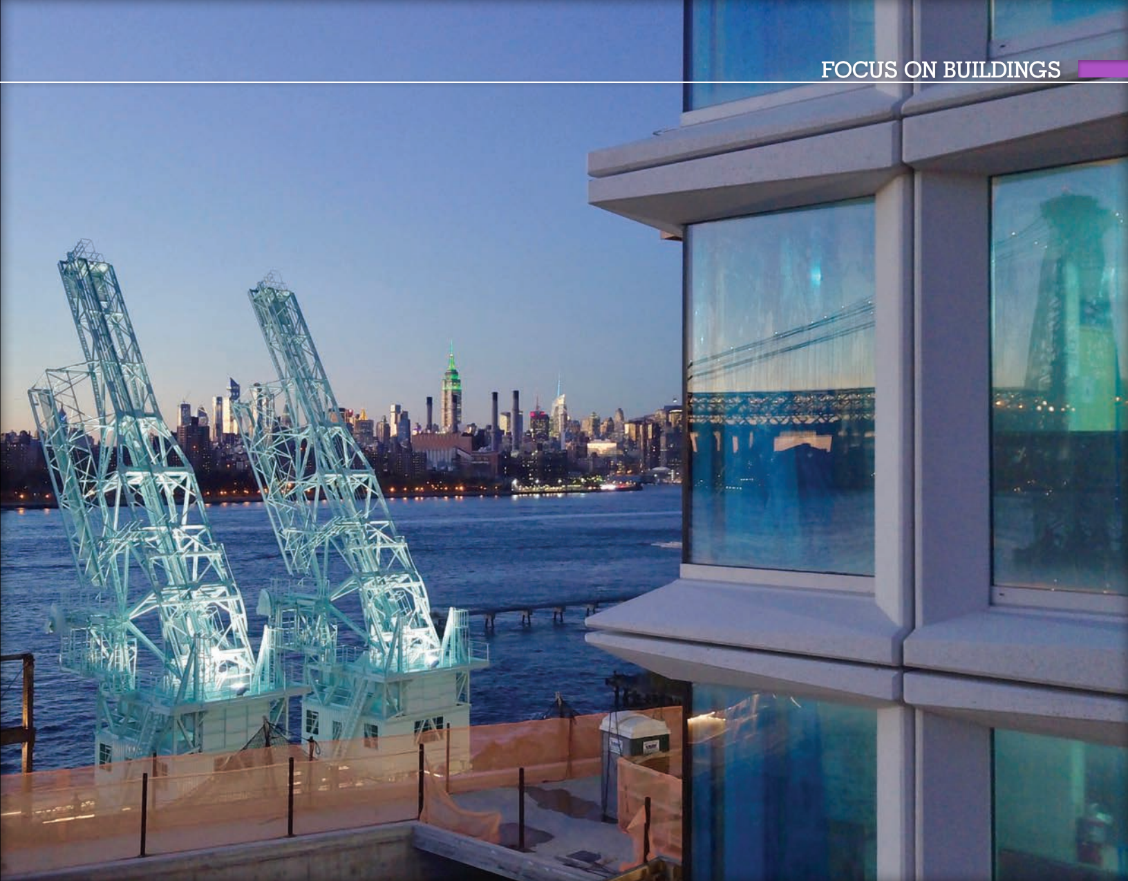
Precast concrete parts, poured from molds developed at ORNL, are installed in a residential and commercial tower on the site of the Domino Sugar Factory along the waterfront in Brooklyn. Windows in the tower resemble sugar crystals. Image credit: Gate Precast
